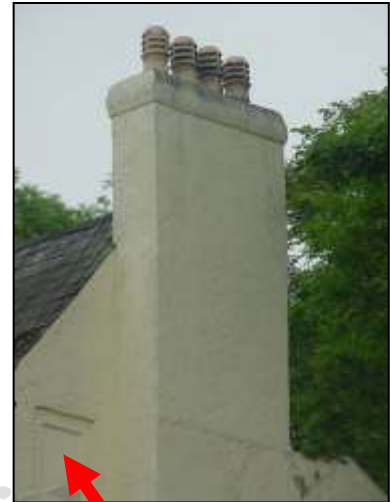
Lean in chimney and door blocked off
