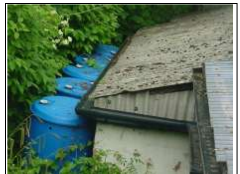
Asbestos roof over the kitchen
