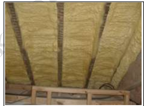
Spray foam in the roof
