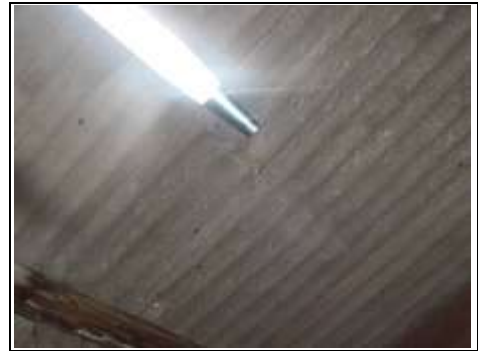
Asbestos roof – the pen identifies cracking in the roof
