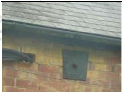
Tie Bar on the back of the function room
