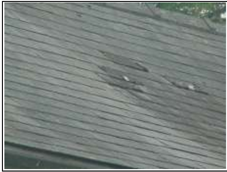
Main roof with some lead tingles
