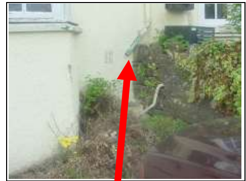
Rainwater discharging onto the wall, leaving the wall damp
