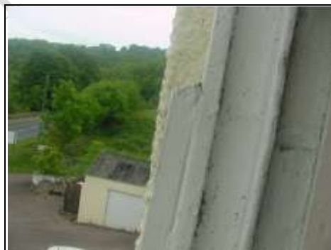
Cover plate over the timber window
