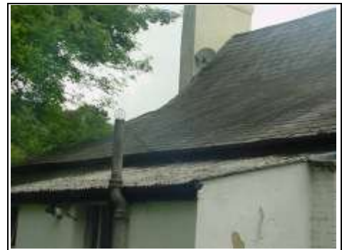
Asbestos roof
