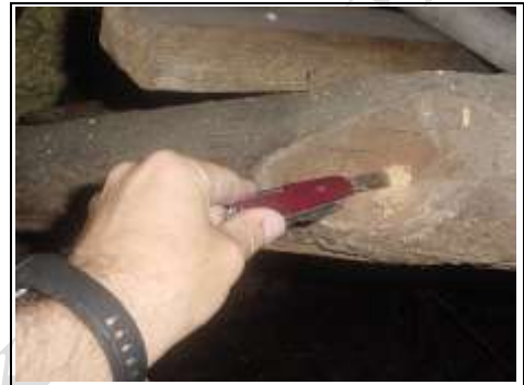
Active Woodworm in the roof
