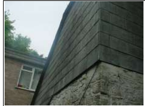
Vertical tiling –rear left hand side
