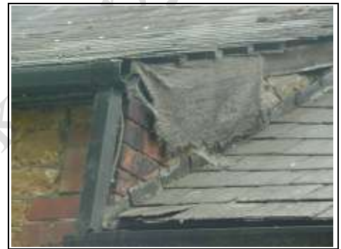
Rear roof where battens are exposed.
