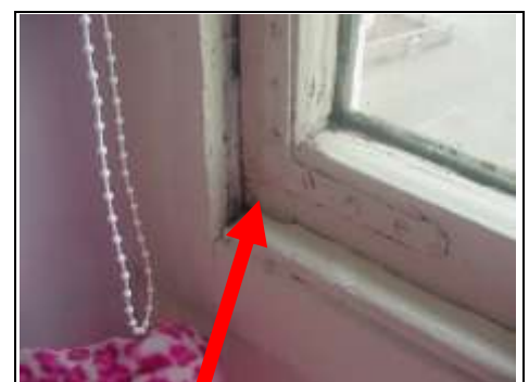
Angle bracket holding the window together on the second floor bedroom
