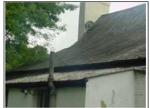
Asbestos roof and flue
