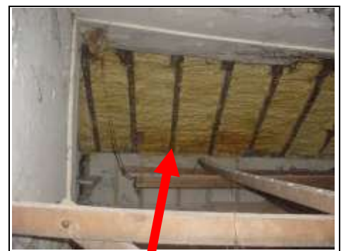
Discolouring could be due to dampness getting in
