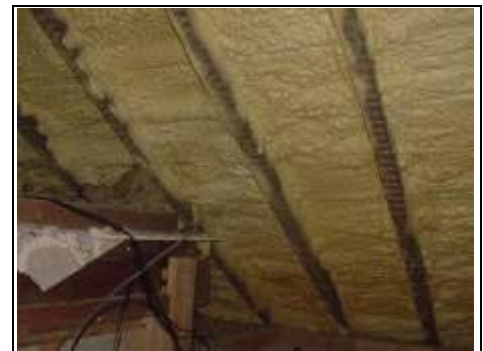
Spray foam in roof
