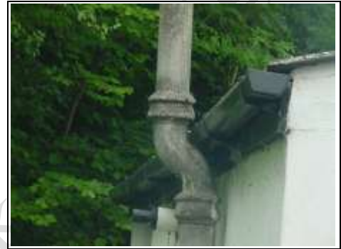
Asbestos soil and vent pipe
