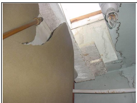
Damp coming through roof window
