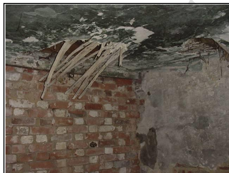
Rear left Room, lath and plaster coming down due to old age and dampness
