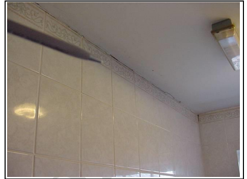
Cracking at high level
