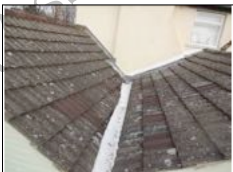
Leaking, painted sealer on top of lead
