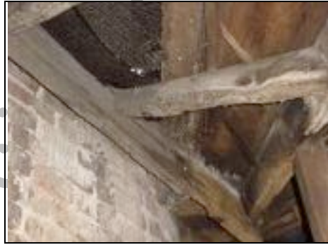
Fire damage/chimney smoke
