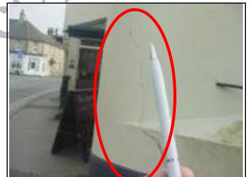
Cracking to right elevation
