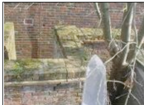
Tree to left causing damage to boundary wall
