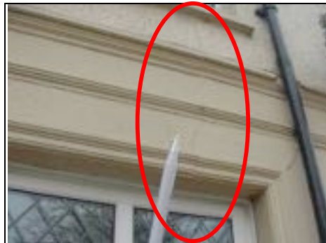
Cracking to right elevation
