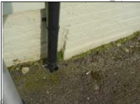
High ground level to rear of toilets and right hand storage area
