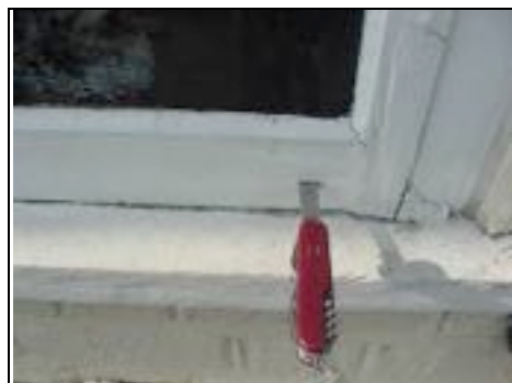
Timber in poor condition
