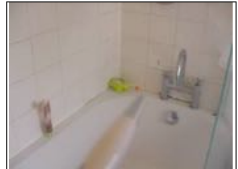
Mould to mastic
