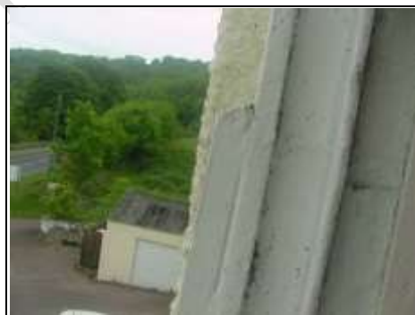
Cover plate over the timber window
