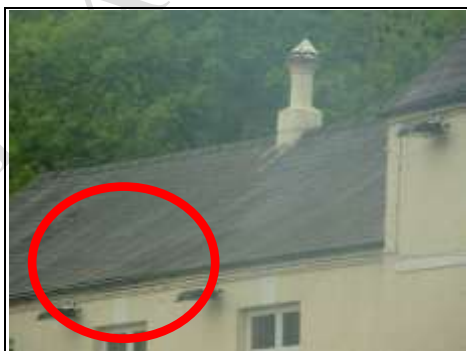
Common rafter feet have deteriorated in the area circled.
