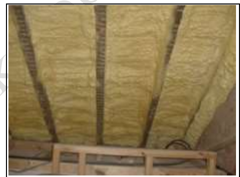
Spray foam in the roof
