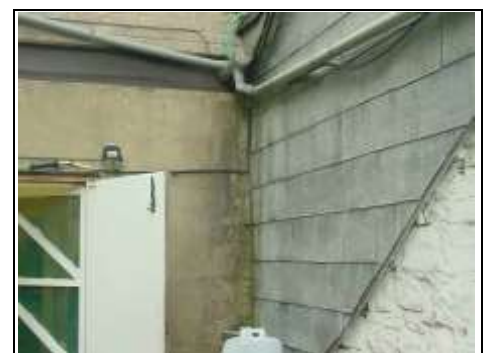
Water overflowing from staircase to function room area
