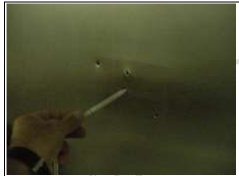
Holes in the stainless steel
