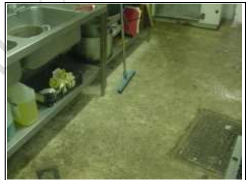
Floor that will not meet environmental health standards
