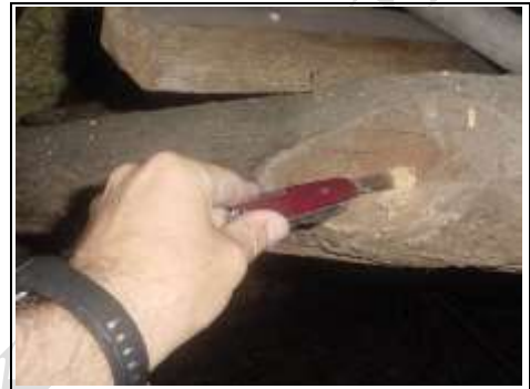
Active Woodworm in the roof
