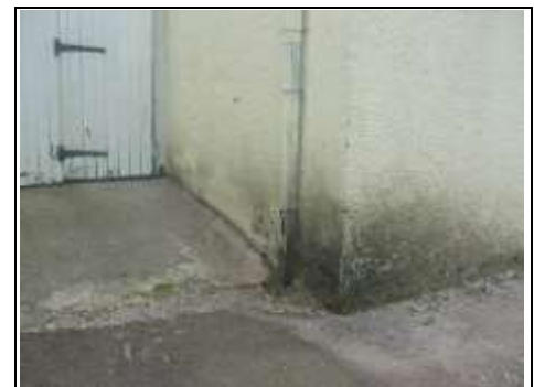
No bell mouth detail to base or render
