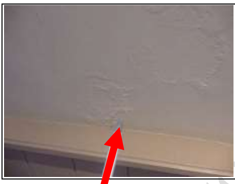
Dampness in front wall in left hand bar
