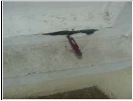
Pushing a knife into the window
