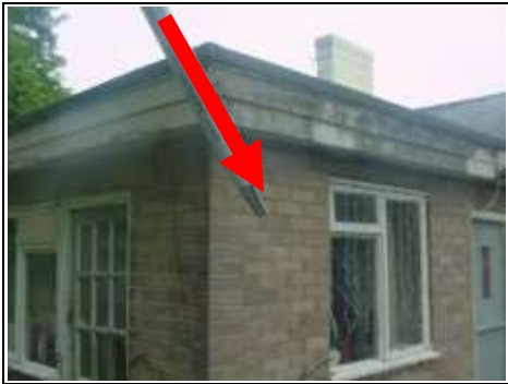
Movement in the stretcher bond brickwork that has been rebuilt
