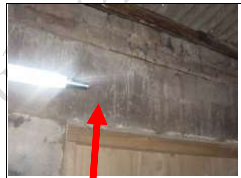
Crack to the lintel in the outbuilding
