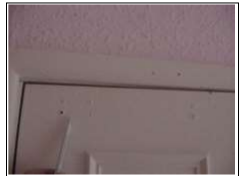
Door closers have been removed
