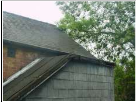
Flashband where the felt roof meets the main building.
