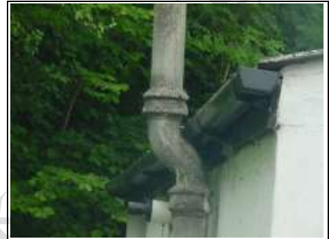
Asbestos soil and vent pipe
