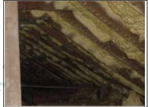
Spray foam in left hand roof
