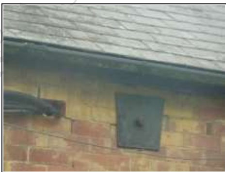
Tie Bar on the back of the function room
