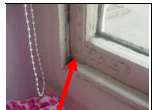
Angle bracket holding the window together on the second floor bedroom
