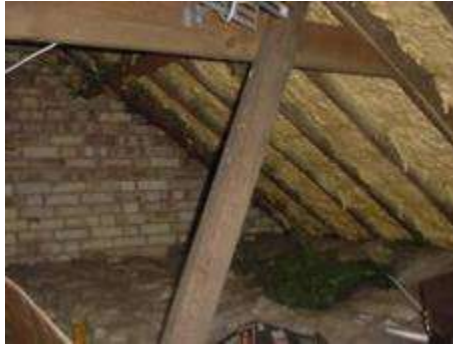
General view of roof with spray foam everywhere
