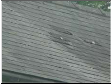
Main roof with some lead tingles
