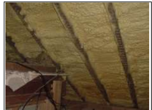
Spray foam in roof
