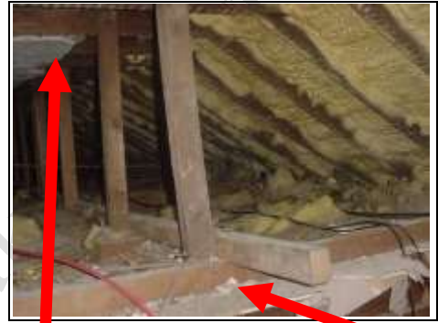
Suspended plasterboard ceiling
