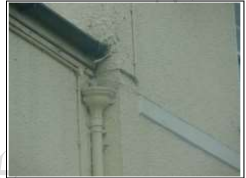
Cast iron hopper head with plastic gutters above.
