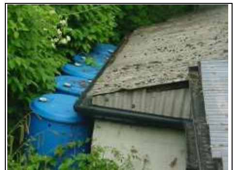
Asbestos roof over the kitchen
