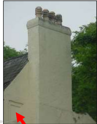
Lean in chimney and door blocked off
