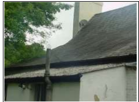
Asbestos roof
