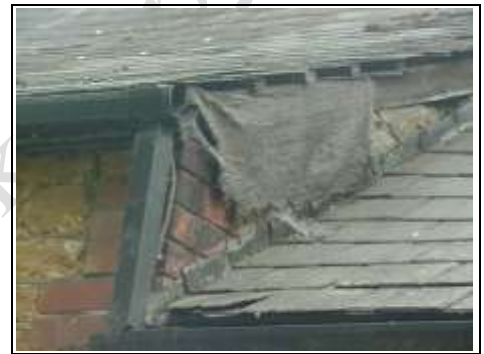
Rear roof where battens are exposed.
