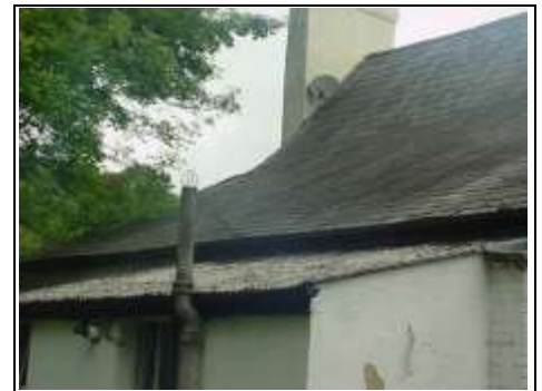
Asbestos roof and flue
