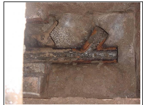
No grease trap present in drains
