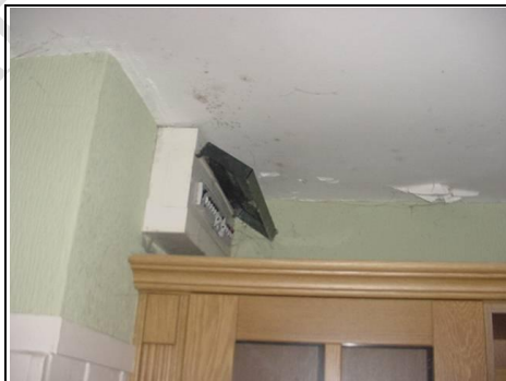
Electric fuse board first floor
