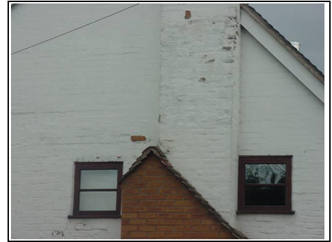
Spalling brickwork
