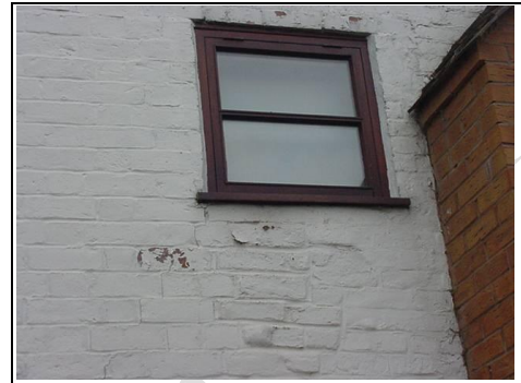
Cracking to corner of window
