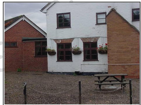
Painted and unpainted brickwork
