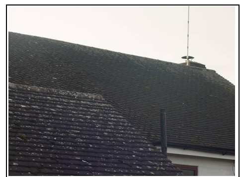
Soil and vent pipe in the centre of the photo
