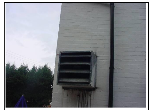
Example of Stretcher Bond brickwork to the right hand side of the property.
