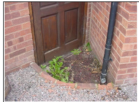
Rainwater discharges and goes through door to cellar
