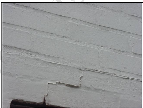
Cracking to Stretcher Bond brickwork
