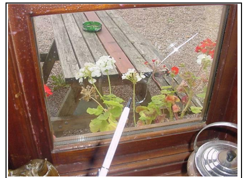
Cracked glass could indicate movement is still occurring
