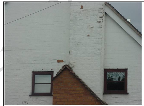
Spalling brickwork
