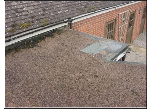
Asphalt covered flat roof to rear with moss
