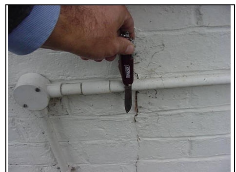
Cracking to rear
