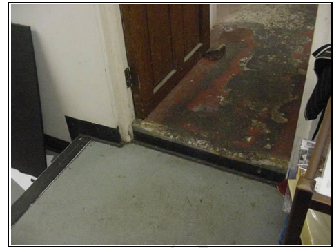
Degrading cellar floor
