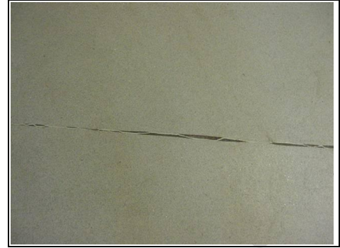
Altro style flooring in kitchen deteriorating
