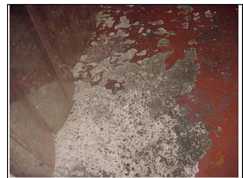
Cellar floor degrading
