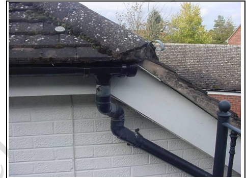
Gutters and downpipes
