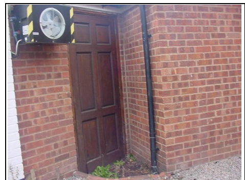
Downpipe allowing rainwater to discharge into cellar
