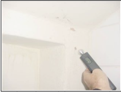
Condensation and dampness getting in relating to valley gutter on right side
