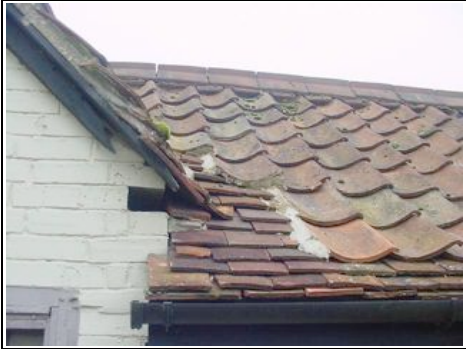
Cement mortar repairs to tiles
