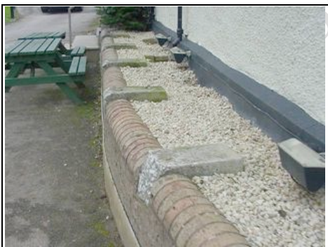
High ground level rather than French drain
