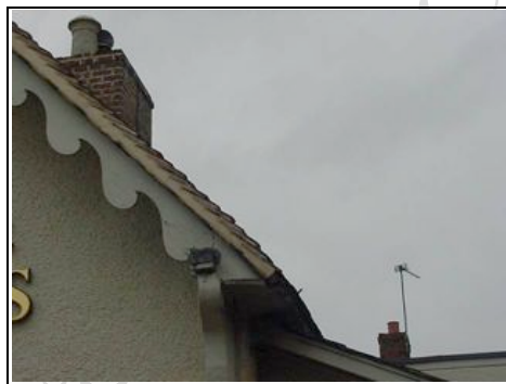
Cement repair to tiles rather than lime
