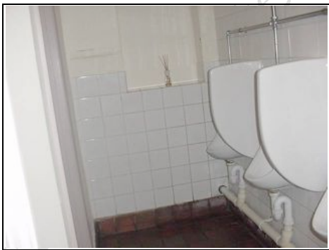
Gents toilets rear right
