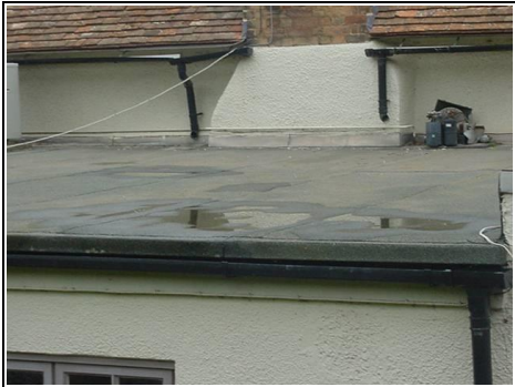
Ponding to flat roof
