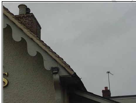
Cement repair to tiles rather than lime
