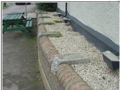
High ground level rather than French drain
