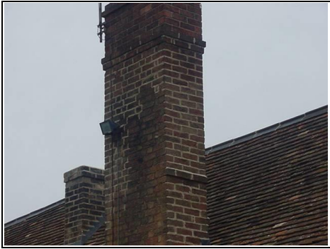
Weathering to chimney
