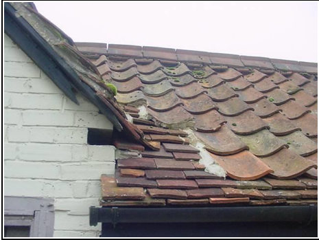
Cement mortar repairs to tiles
