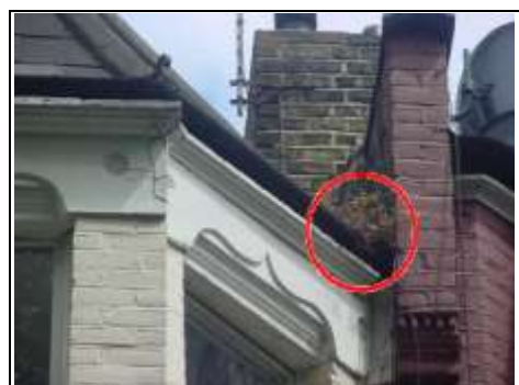
Valley gutter blocked
