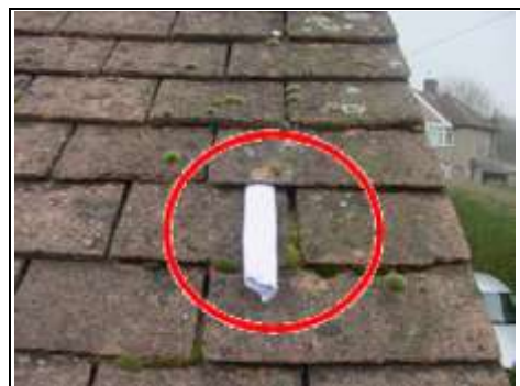
Signs of movement in roof
