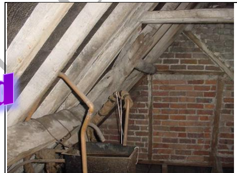
Dampness to wall between front and rear roof
