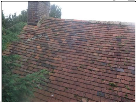
Deterioration to tiles
