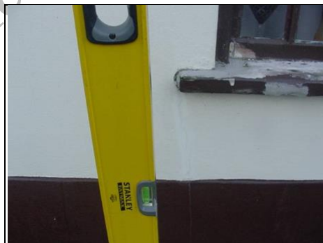
Cracking below window
