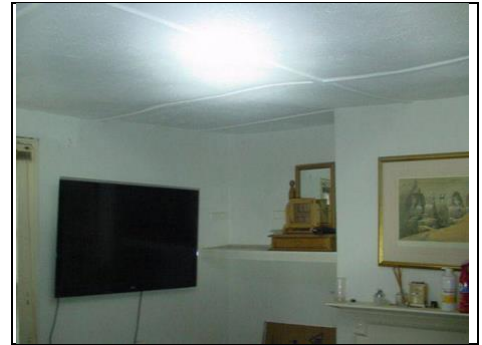
Undulating ceiling
