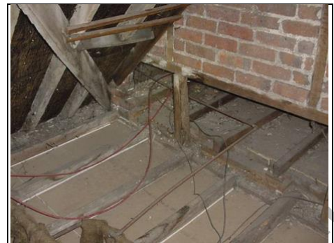
Dampness particularly to roadside end
