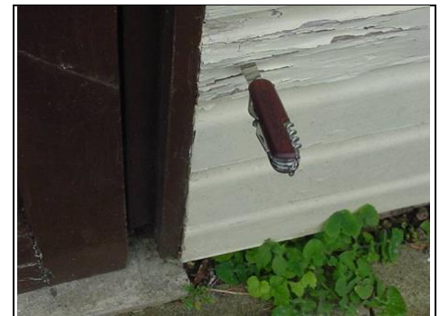
Wet rot to horizontal cladding to rear
