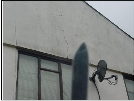
Cracking above metal window to rear of building
