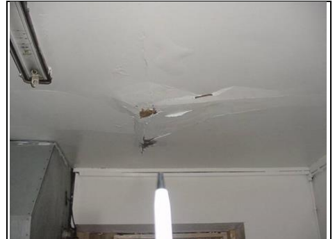
Staining and undulating ceiling in catering kitchen
