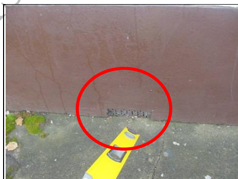
Airbrick acting as gutter
