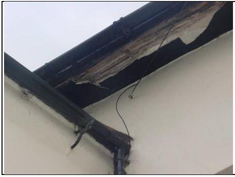
Fascias and soffits in poor condition front right building
