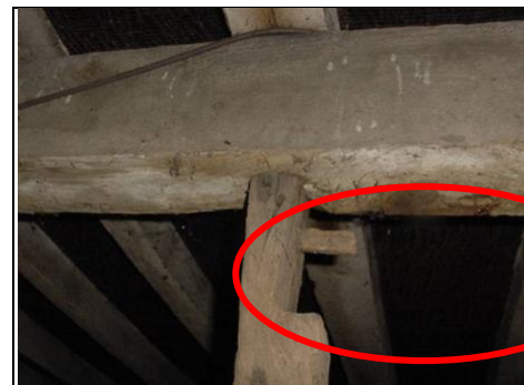
Struts giving support to purlin have been cut
