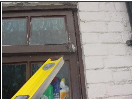
Joints opened up and window falling apart to right
