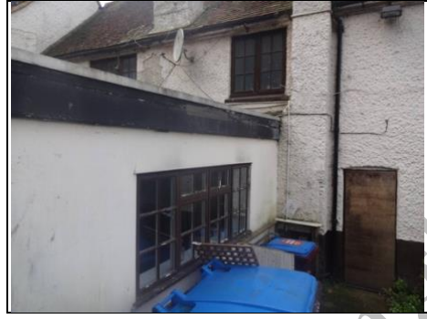
Flat roof fascias and soffits in poor condition
