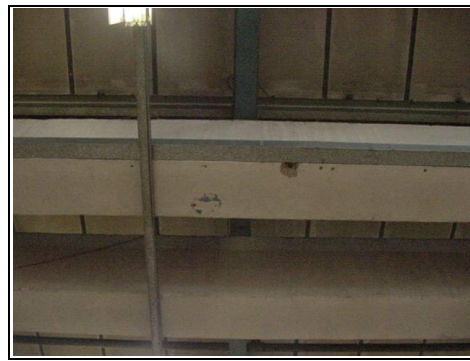
Leaking central box gutter
