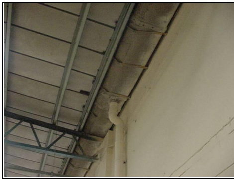
Internal box gutter
